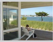
deep overhangs on eastern and southern exposures shield the commons from harsh sunlight and provide welcome shade for study and thought the building blends with the natural environment and enhances the visual impression of Pivers Island from water and town perspectives
